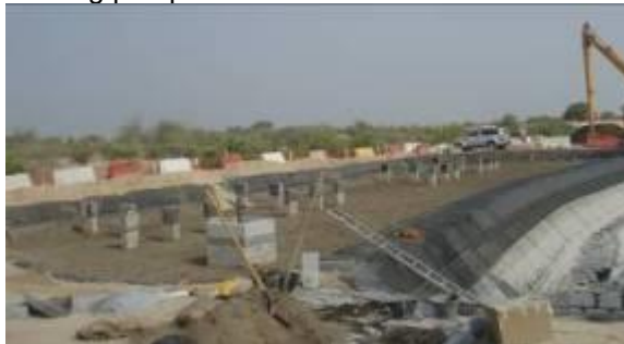
Sand filling of basins
