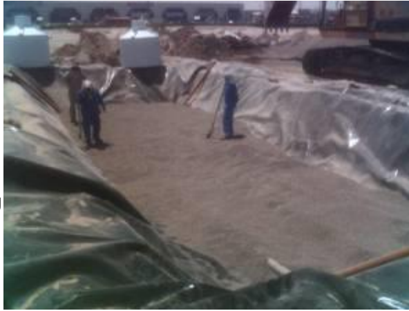
Filling of filter material
