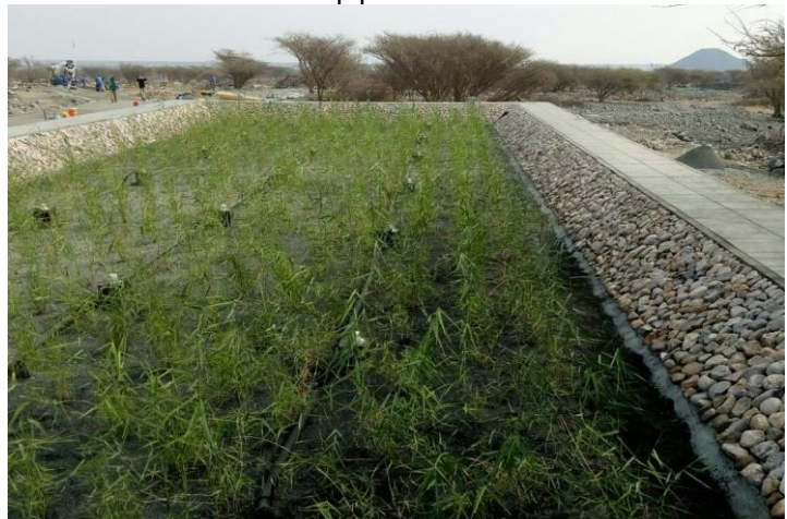
Reed Bed under start-up
