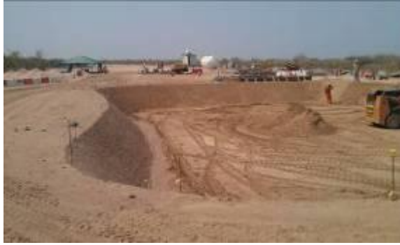
Excavation of basins
