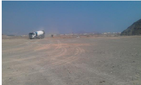
Start of excavation and filling
