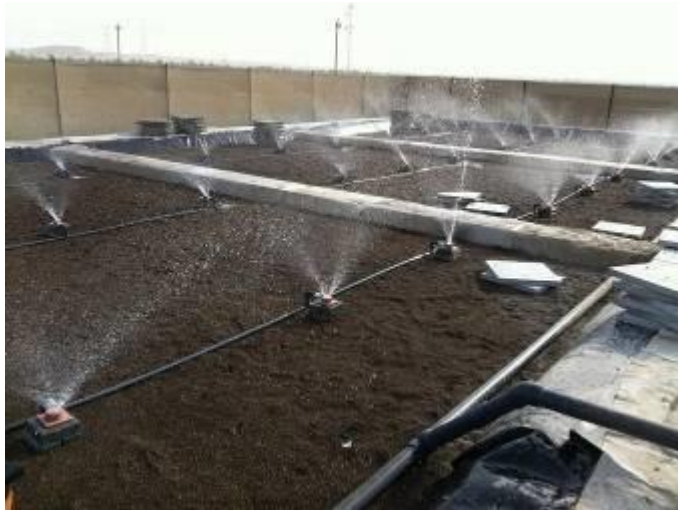
Spray nozzles test Stage B
