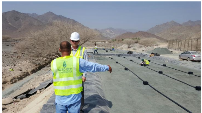
Installation of distribution pipes
