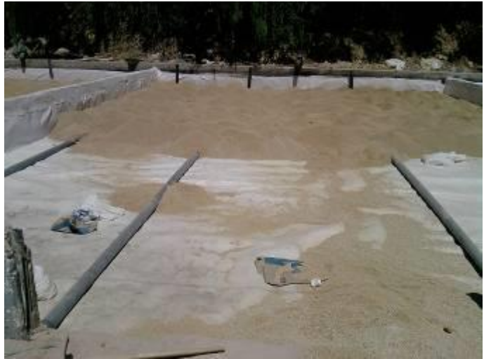
Filter layer installation
