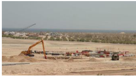
Excavation of pump station
