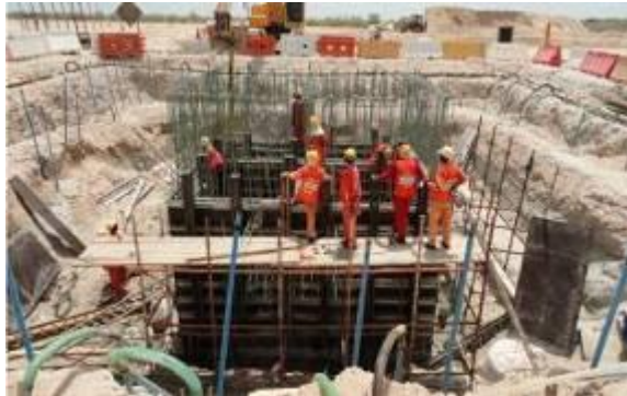
Casting pump station
