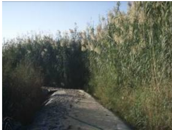
Reed Bed after 1 year of operation
