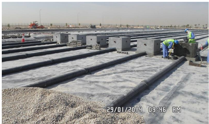
Drainage system and gravel filter
