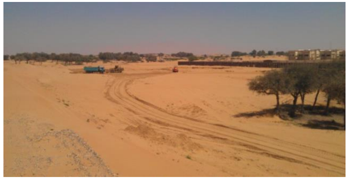
Start of excavation and filling
