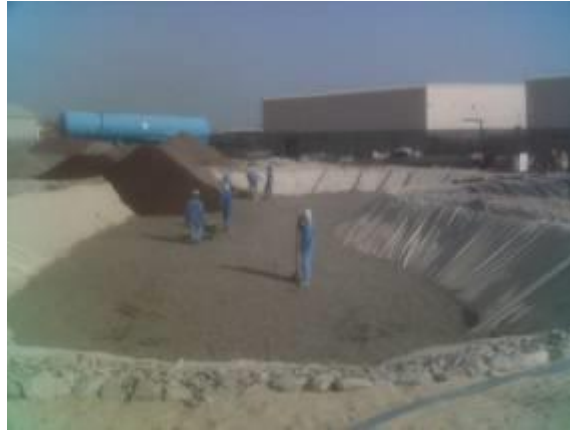
Filling of filter material
