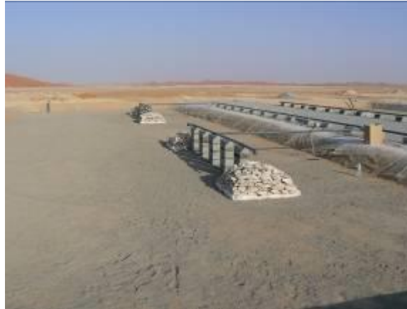
Reed bed 1. stage, under construction
