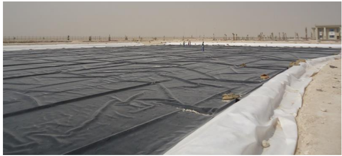
Liner installation
