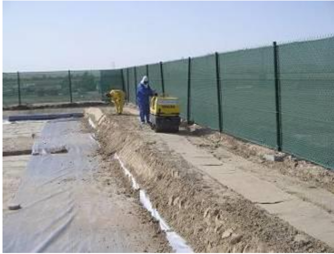
Installation of dams
