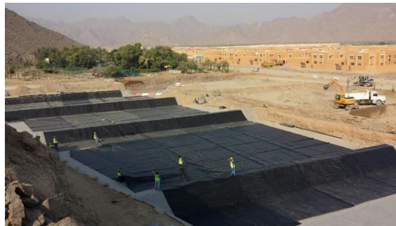
Liner installation
