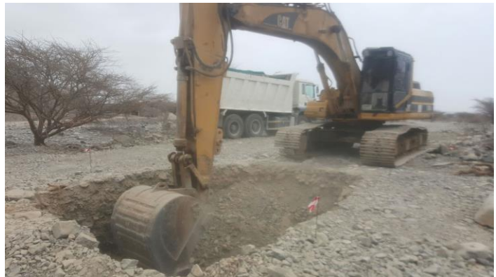
Excavation septic tank
