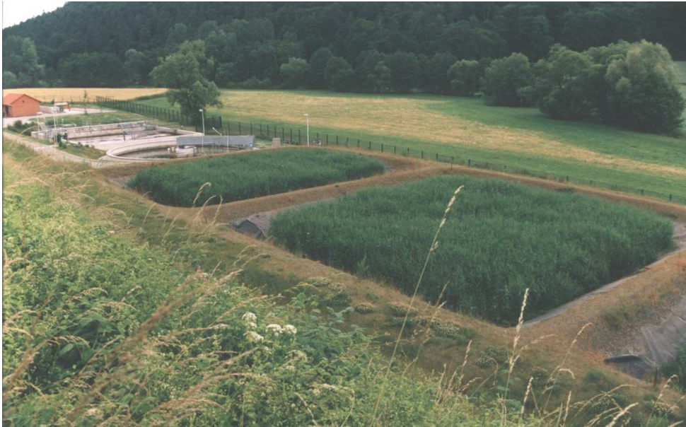
Reed bed dewatering in Naumburg, beds 1 and 2, activated sludge treatment plant in the background
